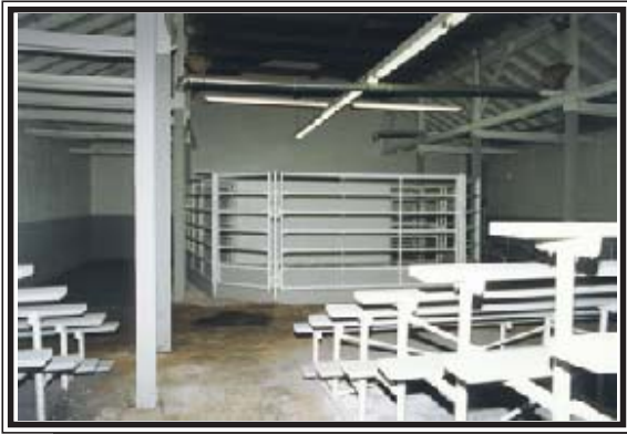
Building 18 Livestock Sale Barn
